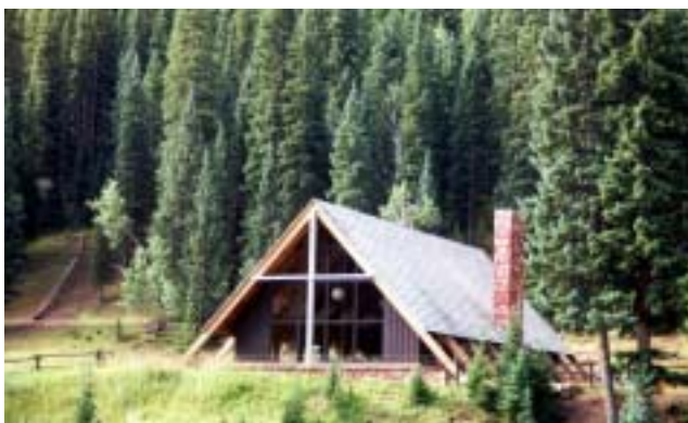
The Chapel with its original wood shingles needs a new roof that is fire resistant and attractive
