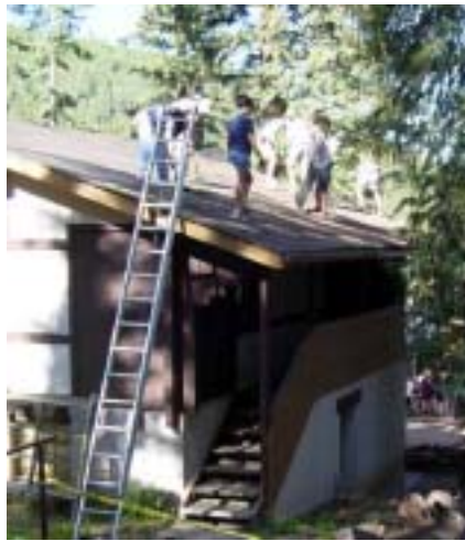
Eiger receiving a new roof this summer
